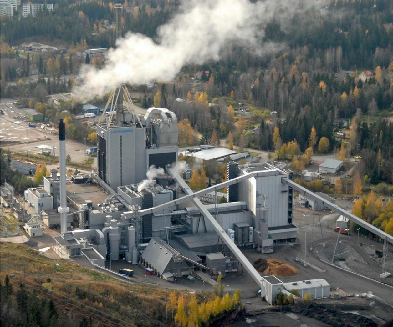
constructed. The automation keeps the electricity and heat generation constant with about 200 guided motors, almost 1,000 measuring points and a price tag of nearly €10 million. In addition to SRF, the plant uses some actual natural gas, e.g., to start up the gasifier, and ignite the burners of the boiler as well as during situations when the plant malfunctions.
